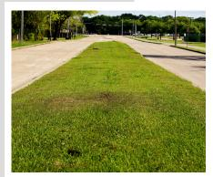
Hydrohay<sup>™</sup> is taking hydroseeding to the next level with almost 2000 kg/ha of conventional mulch and an additional 1500 kg/ha hay providing a solid barrier between the soil and the erosive nature of the environment increasing the critical shear values of the soil by 350-380%.
